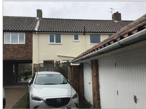
Photo - 2 Rear elevation
