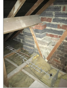
Photo - 7 Purlin built into party wall
