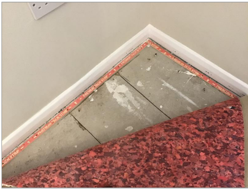
Photo - 10 Chipboard flooring
