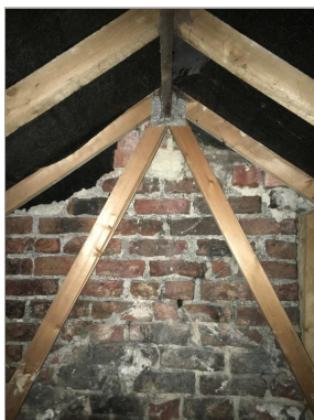
Photo - 4 Roof structure
