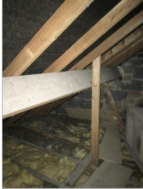
Photo - 6 Purlin and strut support
